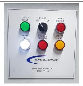
Switch power on via main isolator. Power on LED will illuminate once active.
